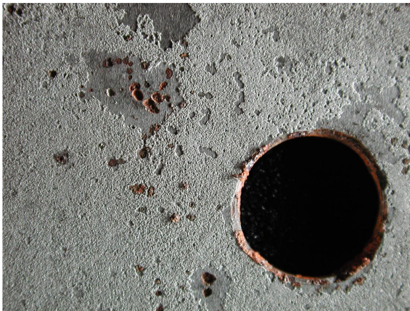
Figure 1 Pitting observed on a 3" × 3" Galfan 200 specimen removed from the Montreal Site after approximately eight years of soil exposure
